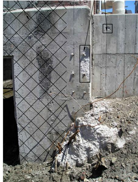
DEMOLISH EXISTING CONCRETE DEBRIS. CORE-BACK EXPOSED REINFORCING STEEL AND PATCH HOLES. SEE (3273) TYP.
