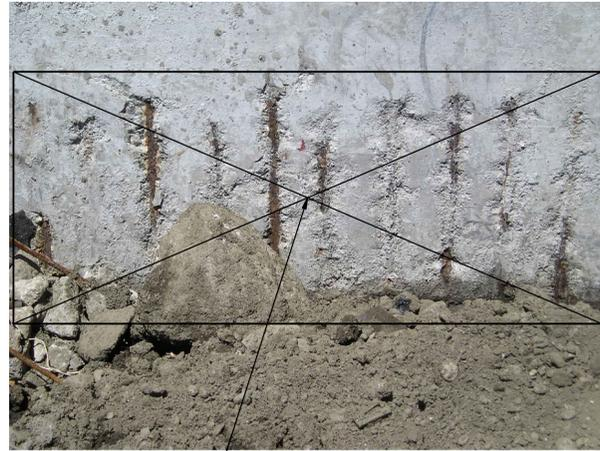
REMOVE UNSOUND CONCRETE, PREPARE CORRODED OR EXPOSED REINFORCING STEEL, AND PATCH CONCRETE SURFACES PER SPECIFICATIONS. TYPICAL THROUGHOUT PROJECT. SEE (3274) THROUGH (3276)
