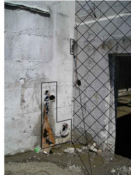
CORE OUT AND REMOVE EXST ABANDONED PIPES AND CONDUITS. PATCH HOLES PER (3271-1) EXCEPT IF HOLES SMALLER THAN 0'-10" PER (3272) SIM.
